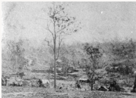
View from Gregory Terrace over what was then known as York's Hollow, 1864 Source: John Oxley Library #108131
