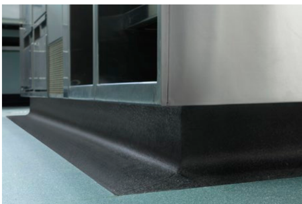
Figure 2: Example of a plinth with coving
