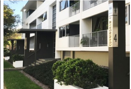
Building entrances are easy to identify and address the street
